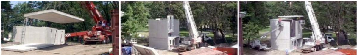
Figure 5: Prefab: Assembly Process
