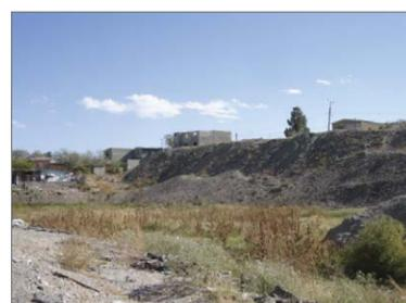
Risk due to eroded slope.
