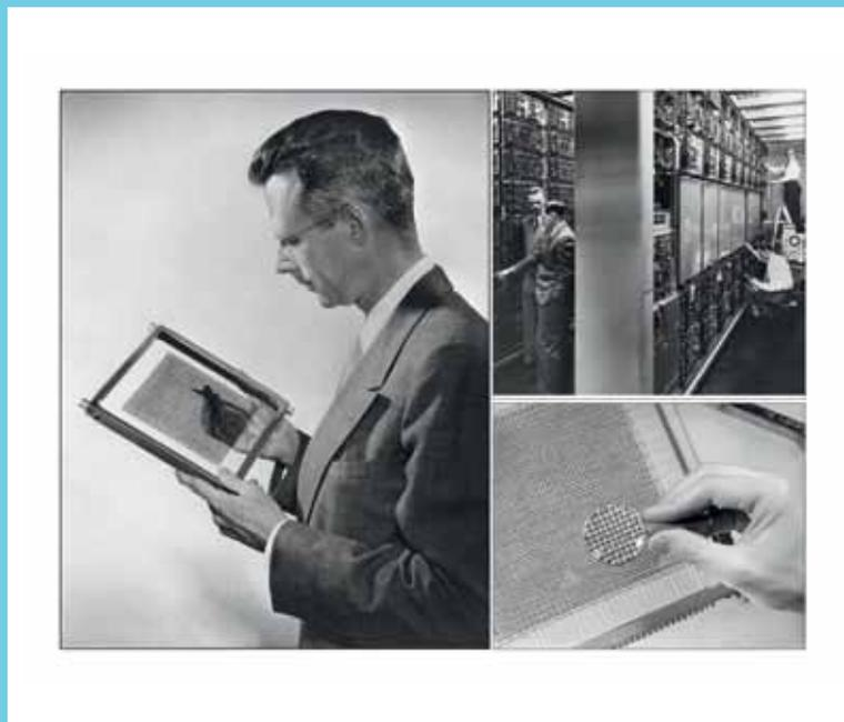
↑ 8. Circuitry: Jay W. Forrester (left) pioneered the development of magnetic core memory (bottom right) and led Project Whirlwind (top right) for the US Navy.
